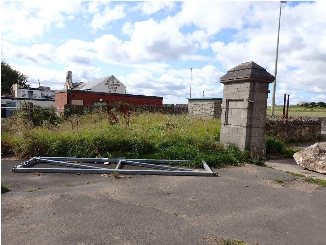
Photo 3: The grassed area to the south of the entrance, with the substation beyond, looking south-west
