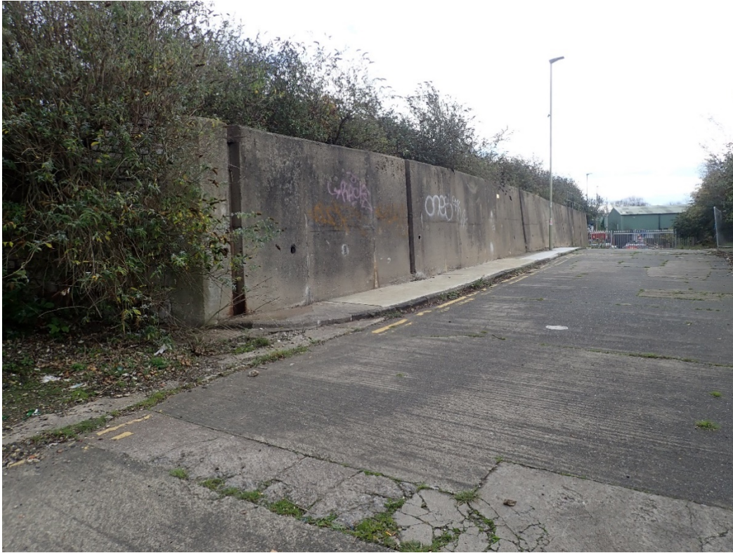
Photograph 5: Concrete wall north of Nile Street, looking east
