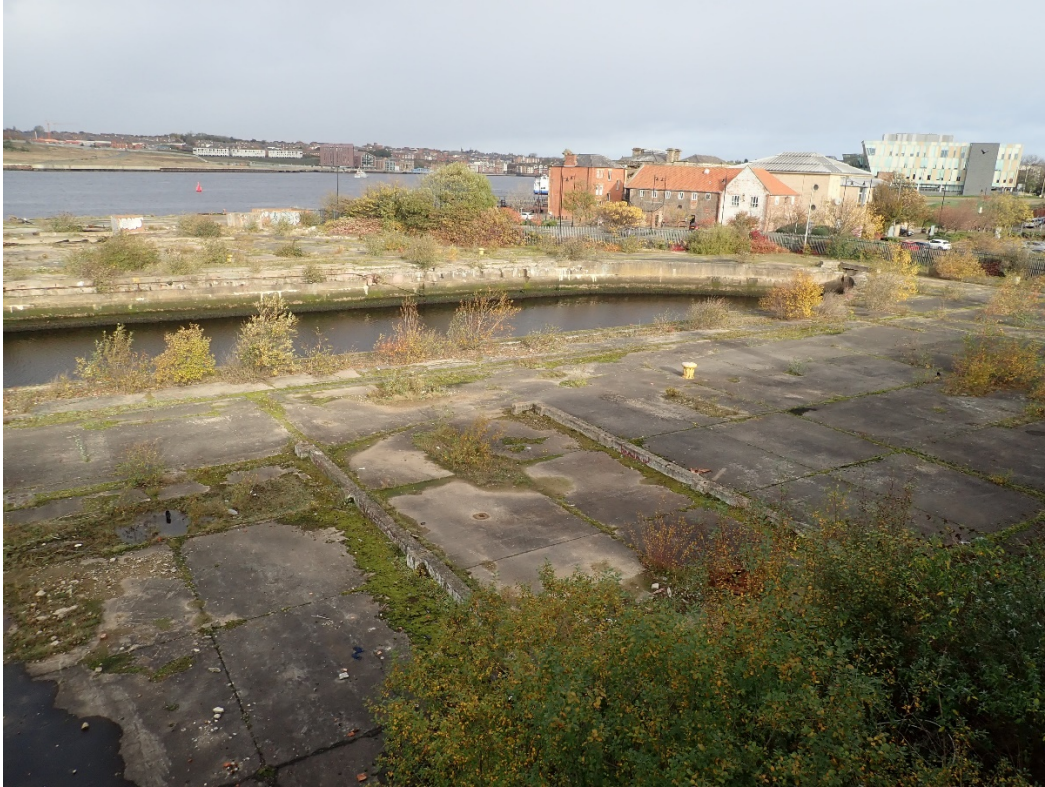
Photograph 3: Northern graving dock, with the Mill Dam conservation area and listed buildings to the north, looking north-west
