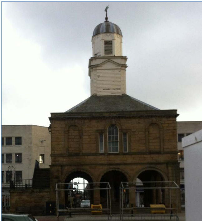
Figure 4.2: West elevation of the Old Town Hall
