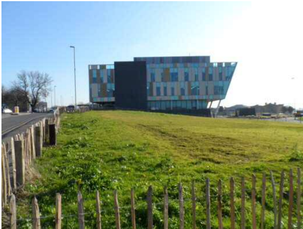
PLATE 8: VIEW SOUTHWARDS ACROSS WESTERN PART OF SITE TOWARDS BT HEADQUARTERS
