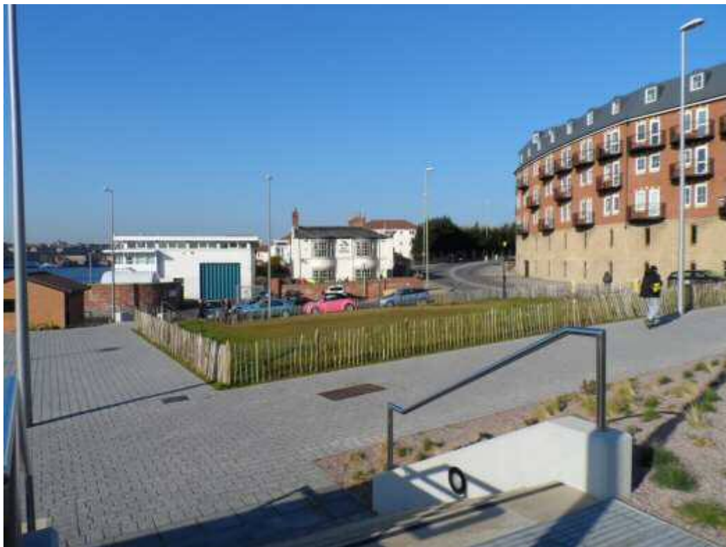
PLATE 9: VIEW NORTH FROM WESTERN PART OF SITE TOWARDS ALUM HOUSE HAM
