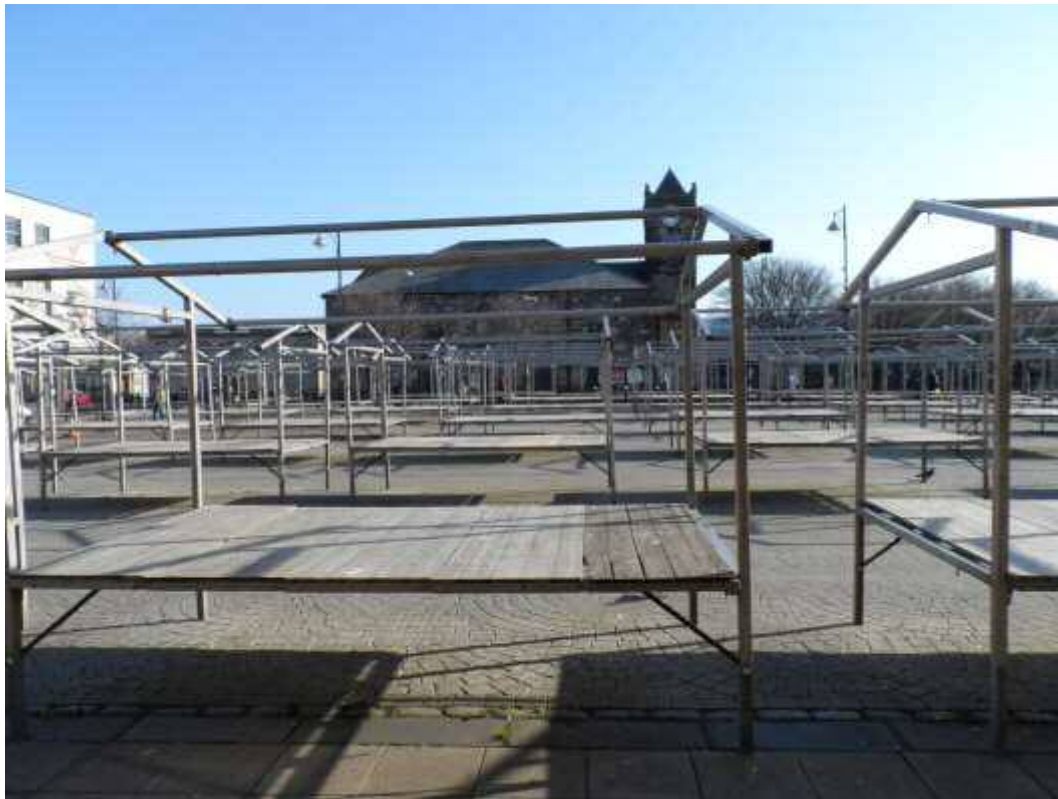
PLATE 2: VIEW SOUTH FROM OLD TOWN HALL TOWARDS THE CHURCH OF ST HILDA
