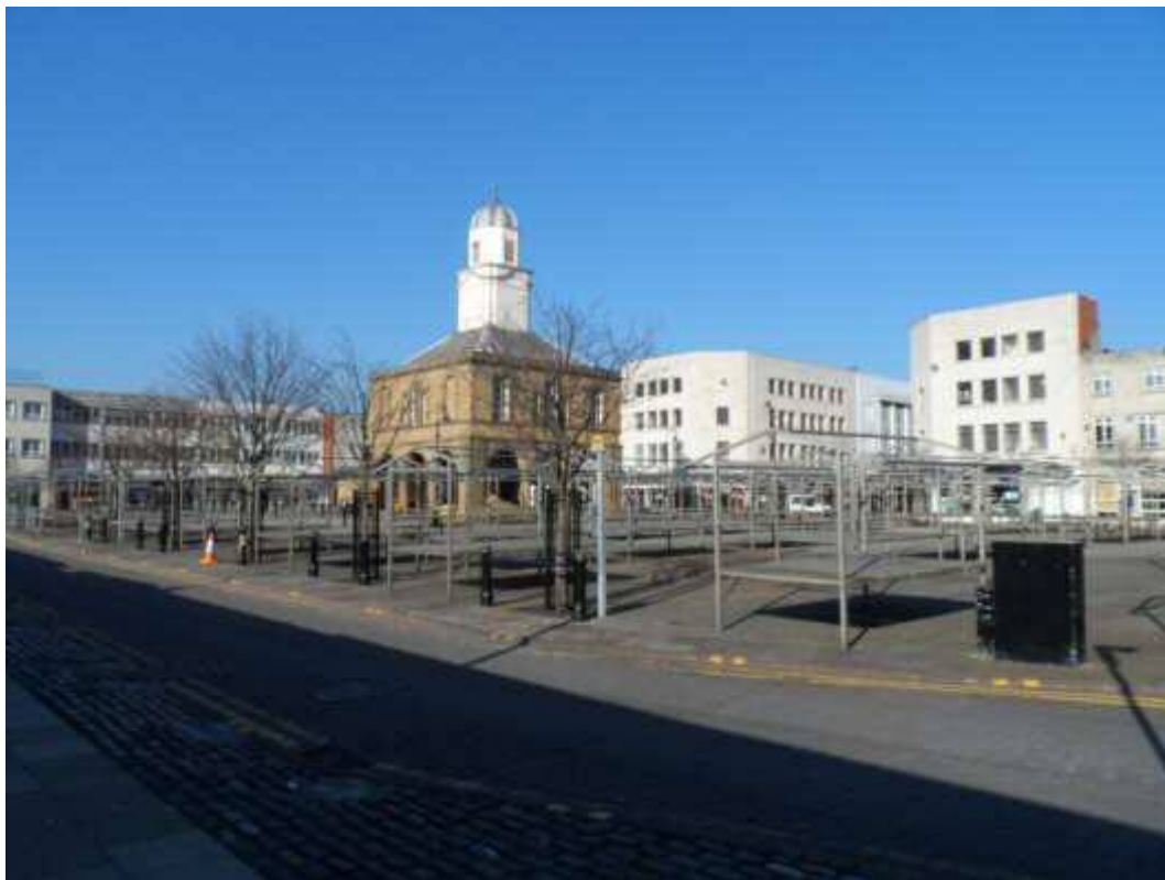
PLATE 3: VIEW NORTH-WEST ACROSS THE MARKET PLACE FROM THE JUNCTION WITH CHURCH WAY
