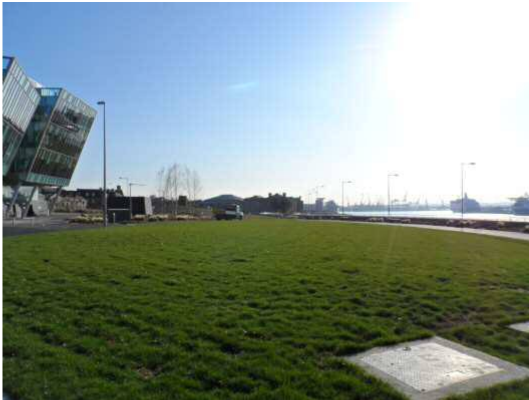
PLATE 10: VIEW SOUTH ALONG THE RIVER TYNE BANK TOWARDS THE SOUTH SHIELDS CONSERVATION AREA FROM THE WESTERN PART OF THE SITE
